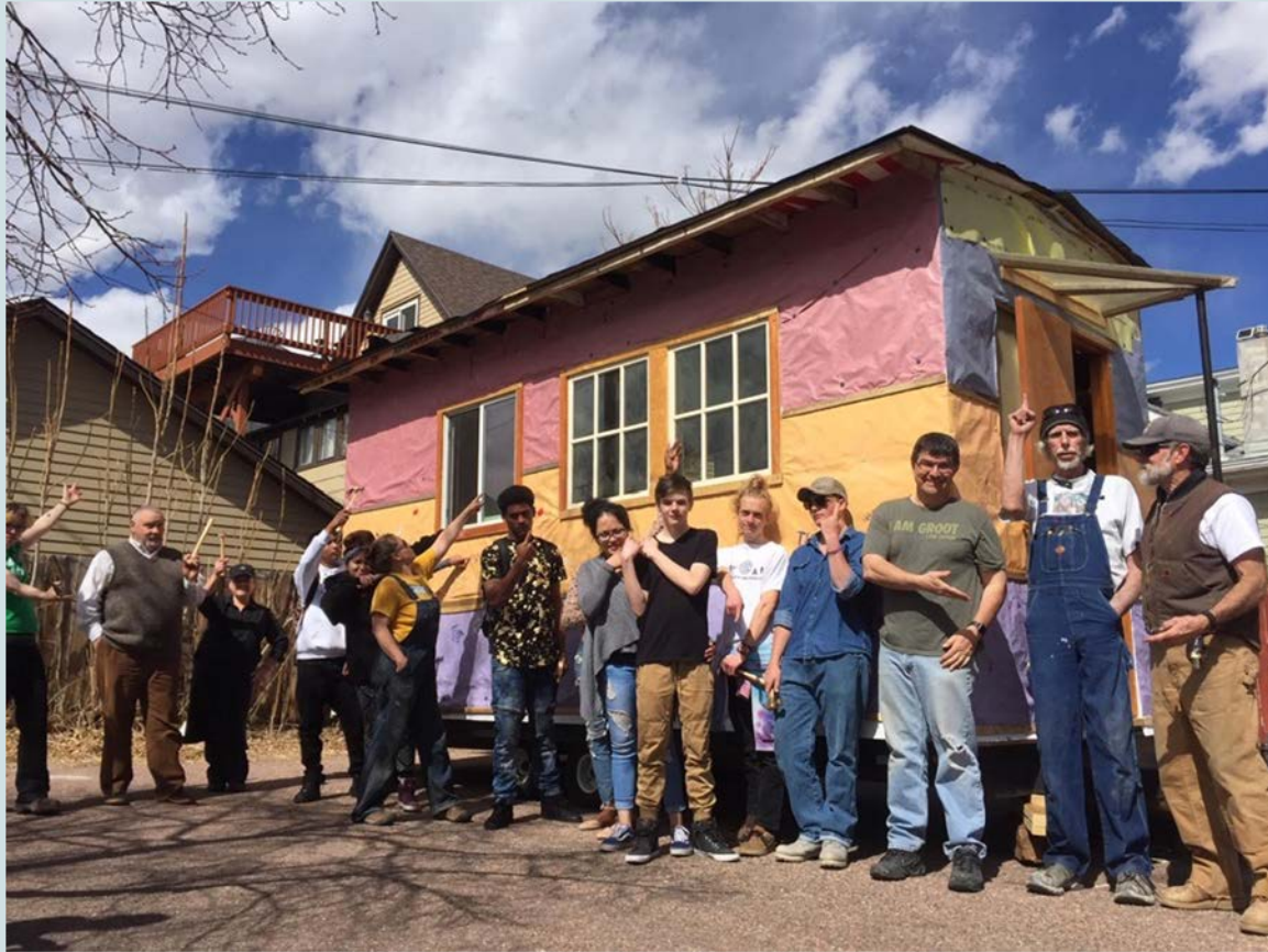
Building the temporary office for Concrete Coyote
