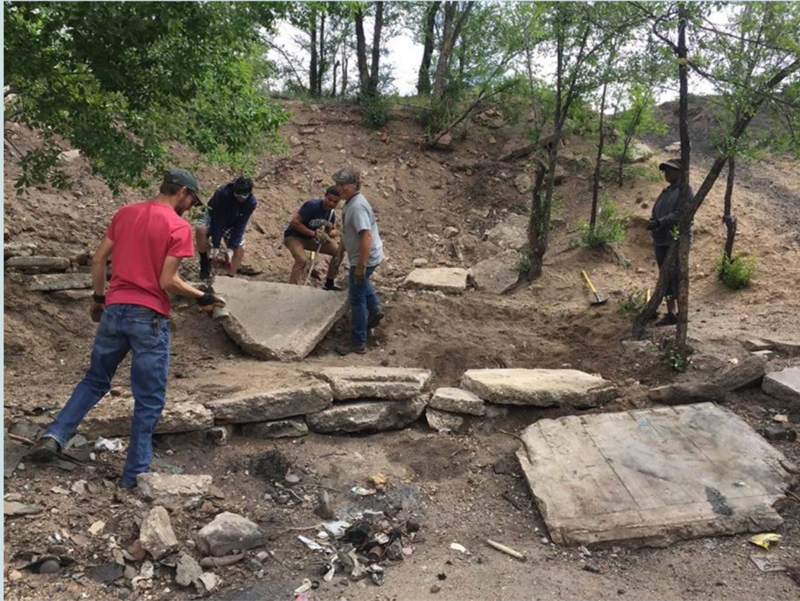
Moving concrete blocks
