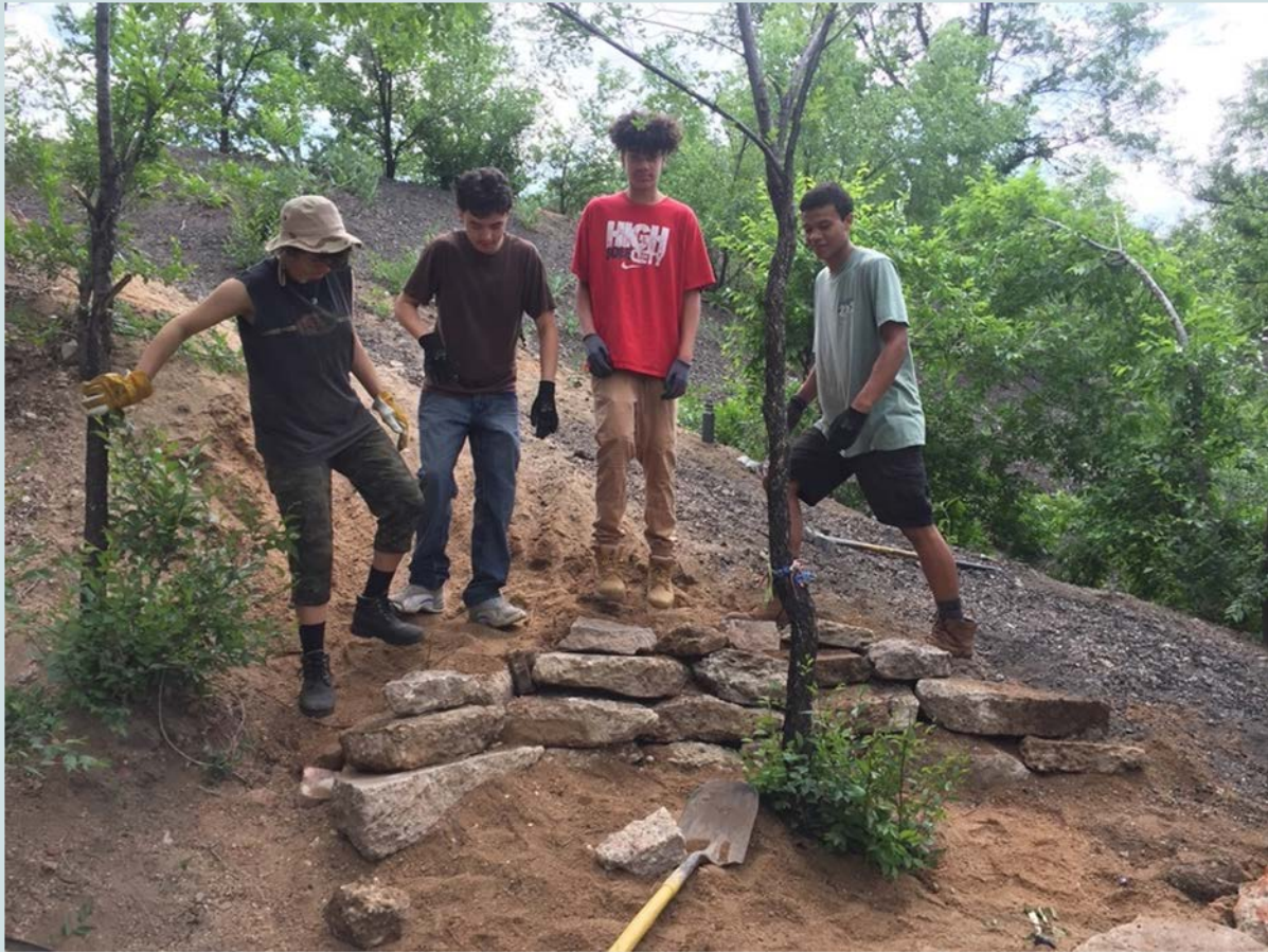
Building a retaining wall
