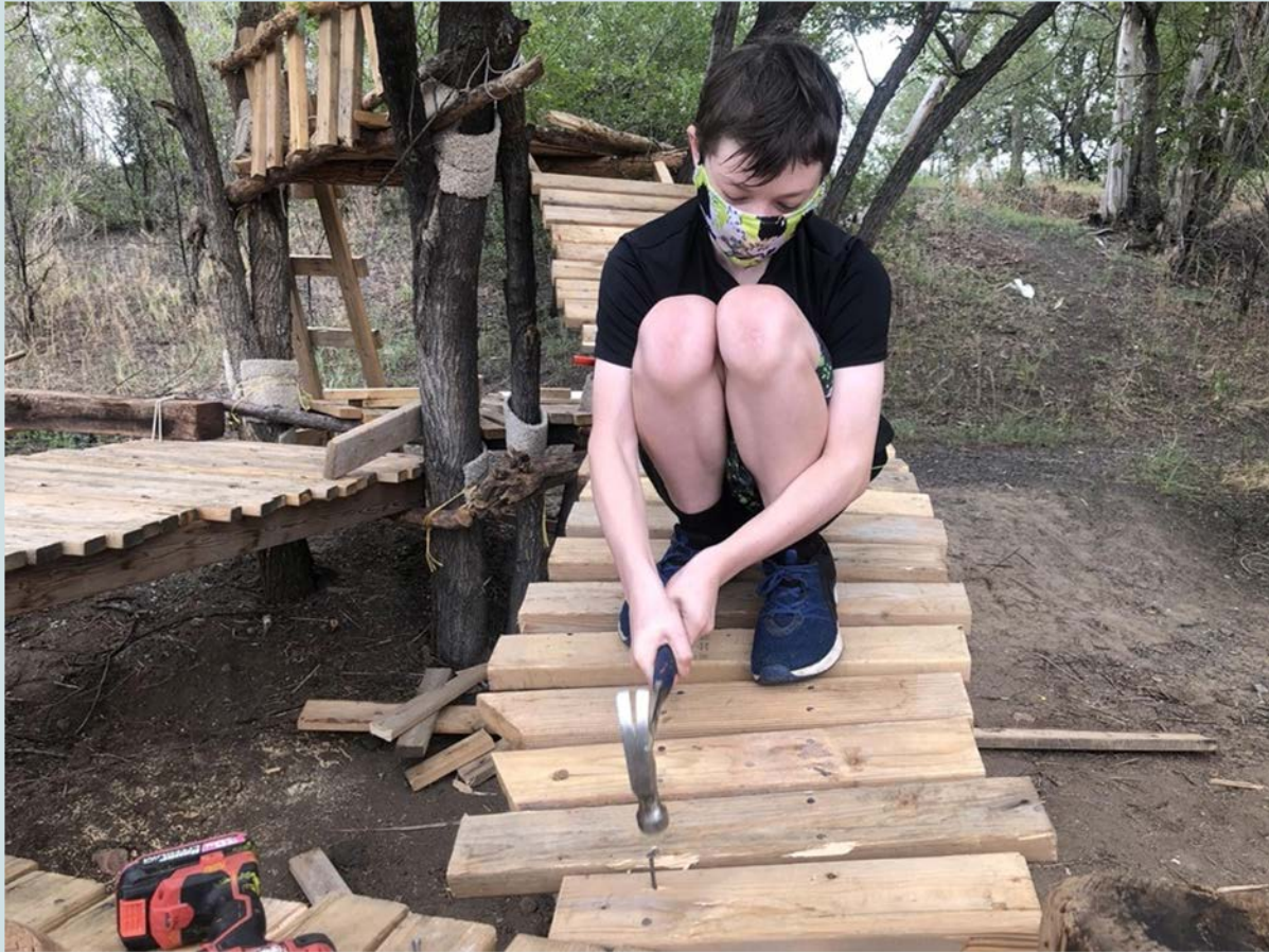
Building the Adventure Park
