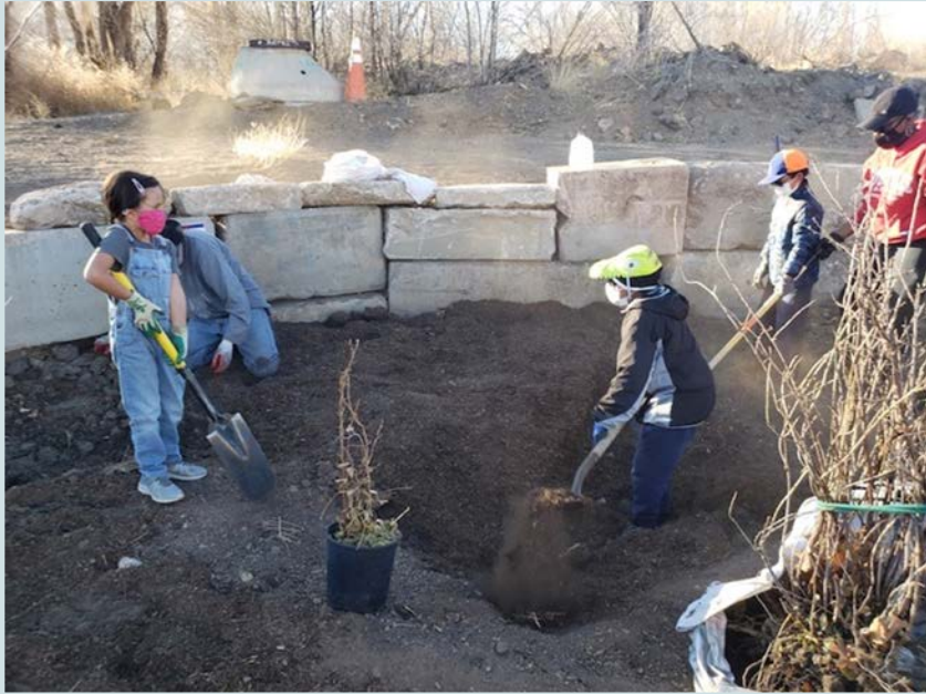
Planting a bioretention swale
